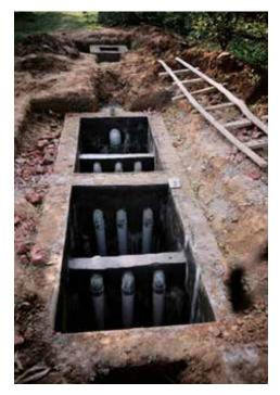
Fig. 2.29: An ABR under construction
