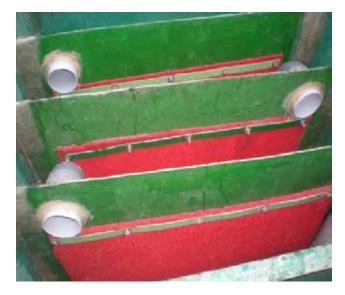
Fig. 2.4 DRDO Biotanks showing different chambers
