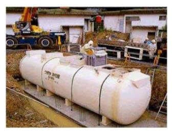
Fig. 2.32: A Typical Package Contact Aeration System (Source: Nishihara Env. Technology, Japan)
