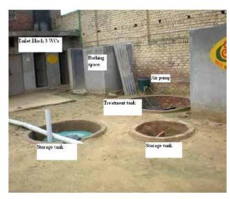
Figure. 2.33 LDDPE made settlingcontact aeration system
