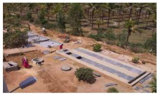
Fig. 2.30. An ABR after completion (http://cseindia.org/content/wastewater-recycling)
