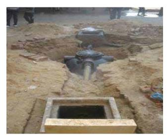
Figure 2.10: A prefabricated Anaerobic Filter installed under Sponsored Project by MDWS (Source Kazmi 2003)
