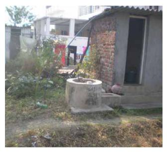
Fig 3.11. A cow dung based biogas plant linked with toilet
