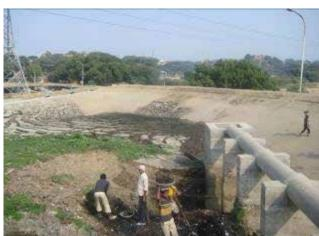
Figure 2.16 Desludging of anaerobic pond (Source: Kazmi 2003)
