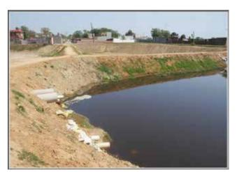
Figure. 2.15 An anaerobic pond of a WSP
