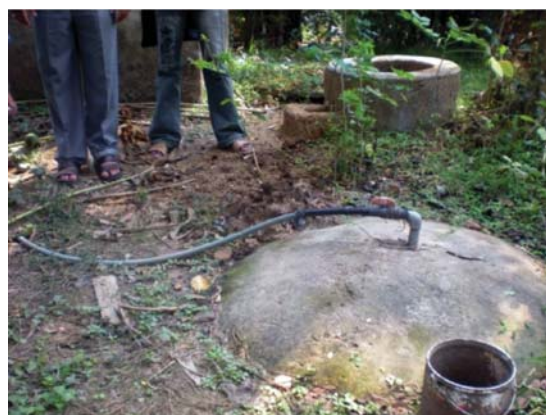
A family size biogas plant
