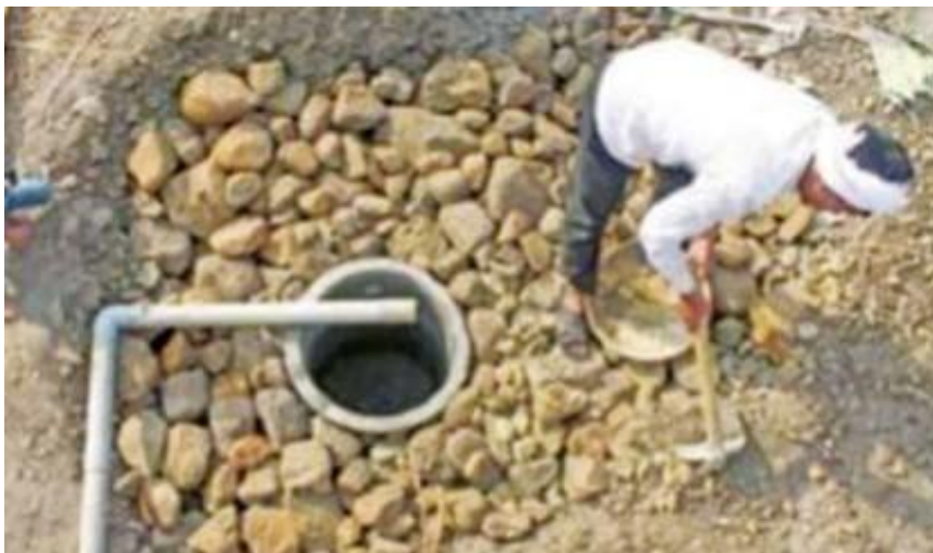
Soak Pit with Earthen Pot
