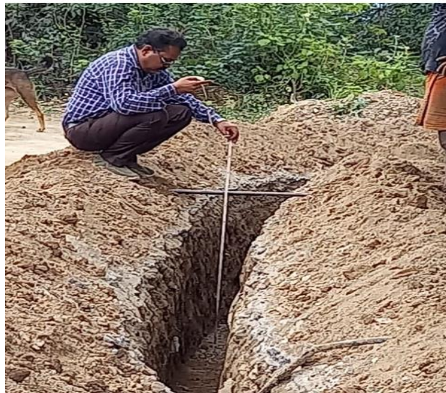
Measurement of trench depth
