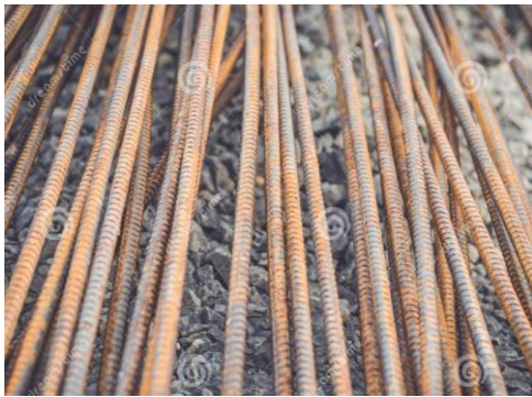
Poor Quality Steel
