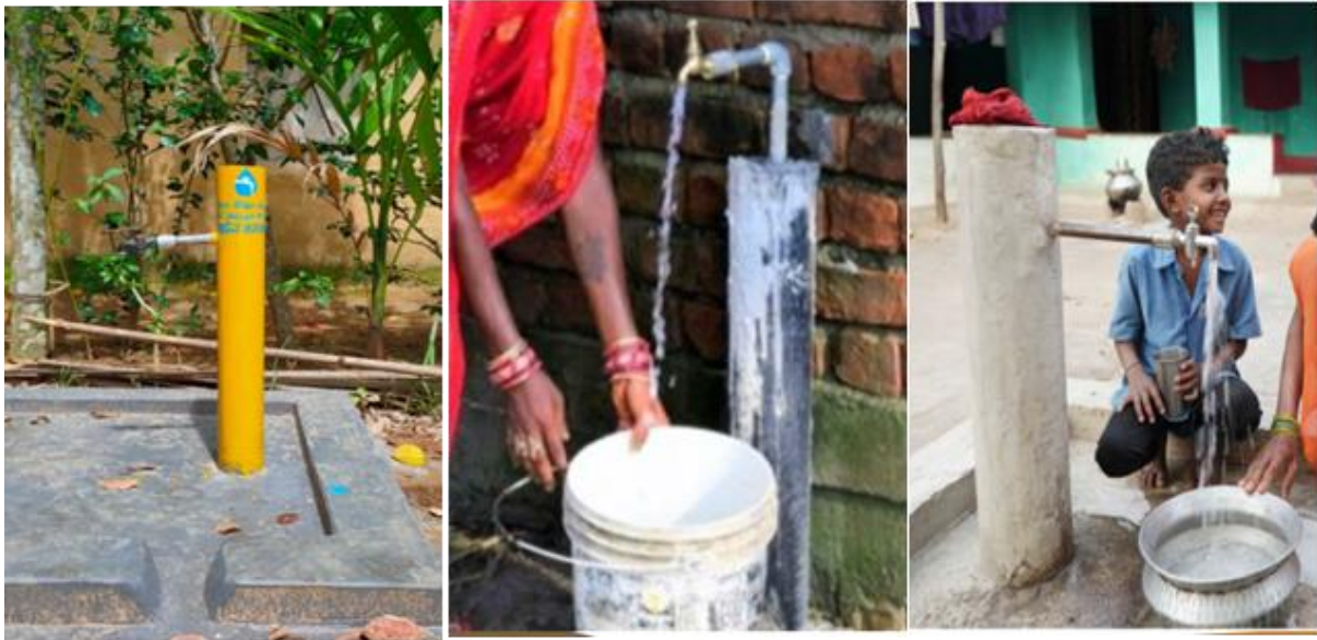
Construction of FHTC – Good Practice
