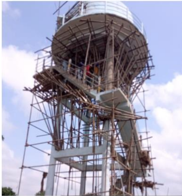
Construction of Overhead Tank
