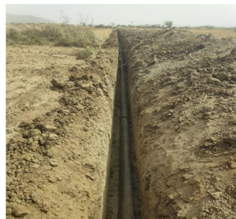
Pipe laying in the trench
